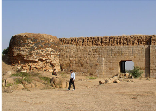
Fig. 5 Exterior view of curtain wall with a mud and masonry parapet in Chittledroog's lower fort; this stretch of curtain joins a round bastion to the left
