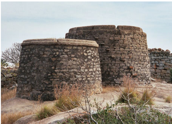
Fig. 9 Two well-preserved masonry granaries at the top of Mergasy’s fortified hill. Access would have been through flat terrace roofs. Slab steps lead up the side of the granary in the background
